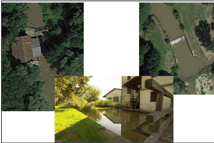
Figure 4: Small Hydropower Plant
