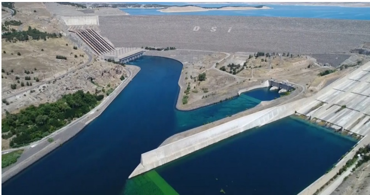
Figure 7. Aerial view of Turkey's Ataturk Dam.
